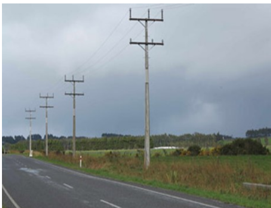
Figure 2: Example of 11 kV distribution line
