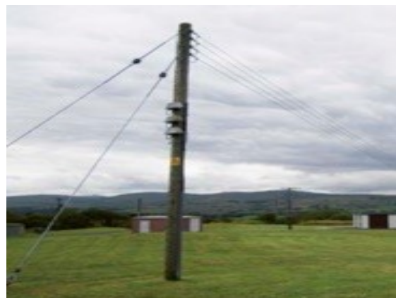
Figure 3: Example of 400 V distribution line
