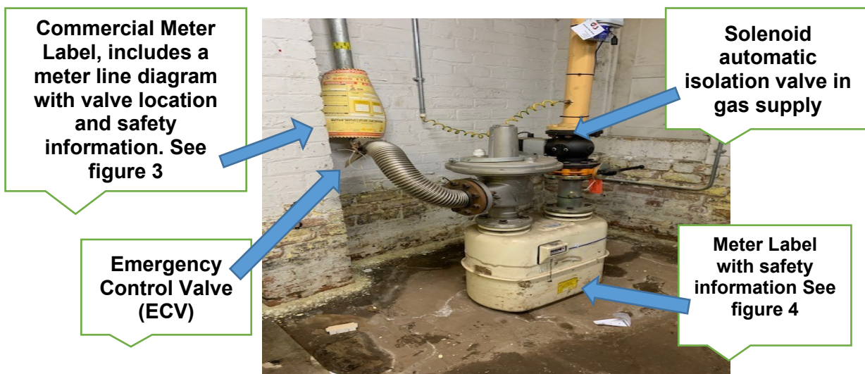
Figure 5: Commercial Gas Meter located in Plant Room
