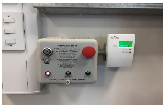
Figure 7: Example of a Gas Proving Unit linked to a CO2 detector
