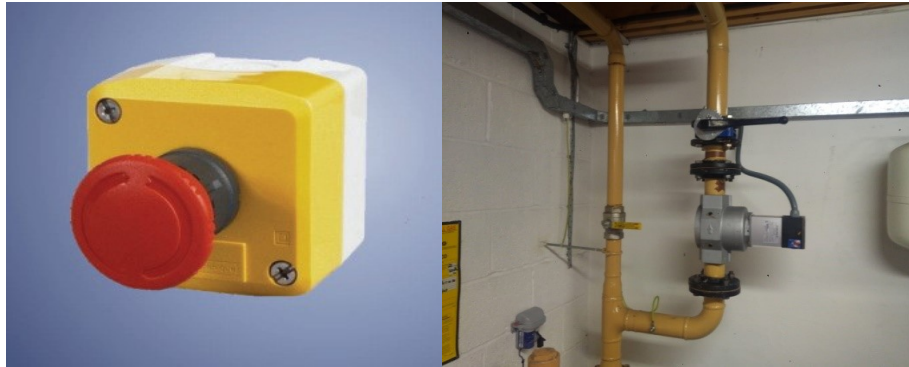
Figure 9: Example of an emergency shut off push button and an automatic isolation valve installed to the gas supply located in the plant/boiler house
