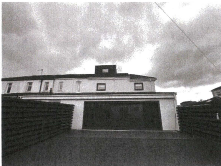
Image 2: Rear of property as built
