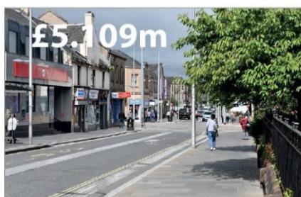
Roads and Footways
