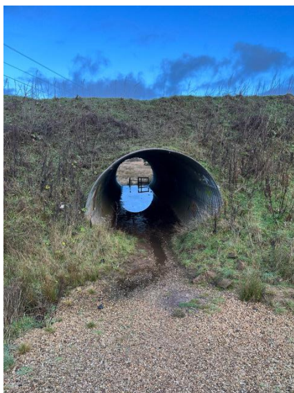
Tunnel on the Clyde Coastal Path outside Milngavie
