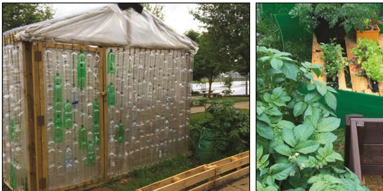
Figure 9: Greenhouse made of plastic bottles and planters at Turnbull High School
